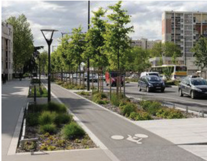
Bio-retention swales
